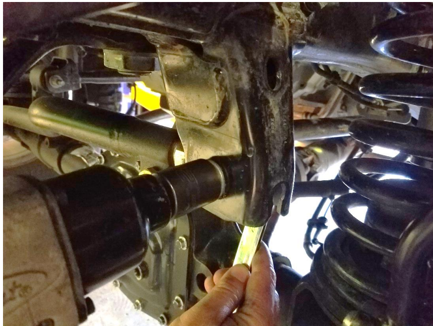
Figure 1. Removing Frame Side Track Bar Bolt
