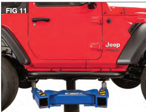
Ensuring that the step is level to the body, slowly tighten the 8mm bolts behind pinch weld on the front and rear mounting brackets. Next, tighten all 6mm hardware so the support brackets are on center with pinch weld holes.
